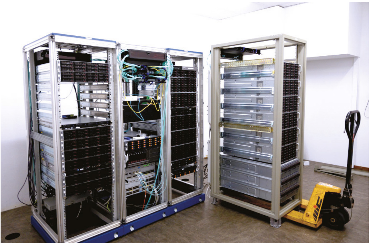
Figure 3.2: Reinstallation of the production equipment after the reinforcement of the raised floor, rotating the racks by 90° to allow for more rack space and improving the cooling air flow. Credit: P. Boven.
