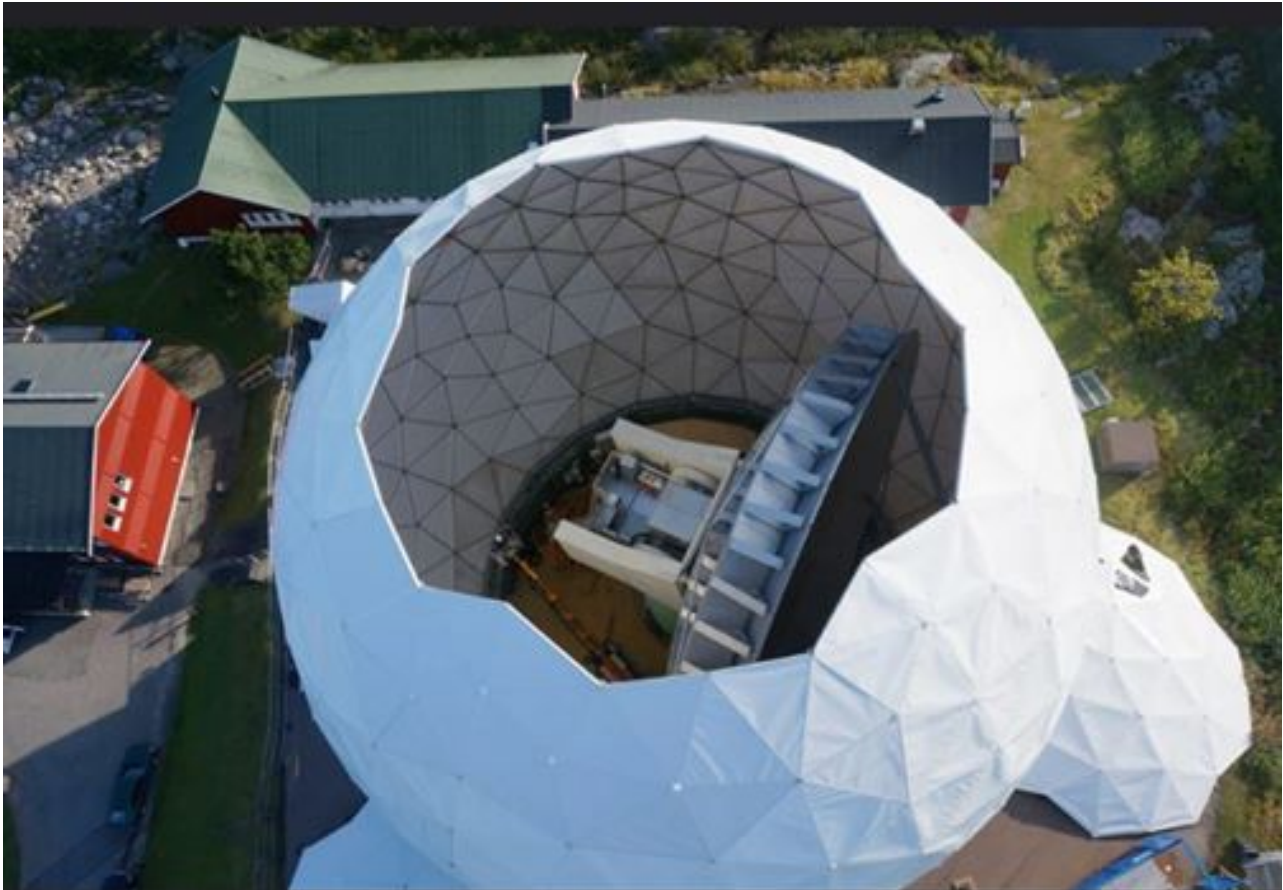
Figure 5. 'First Light' for the Onsala 20m telescope. The original radome (built 1976) of the Onsala 20m diameter telescope is in the process of being replaced. This picture, from 26th August, was taken during the critical operation of replacing the zenith cap. Since the telescope panels were assembled after the erection of the radome in 1976, these few hours represent the first time the telescope has been exposed to the open and hence the 'first light' of the telescope. For more pictures see https://www.flickr.com/photos/onsala/sets/72157646515111850 . (Image and caption credit: John Conway, Onsala Space Observatory).
