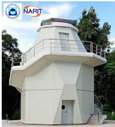
Current at TNRO, Tower by NARIT
