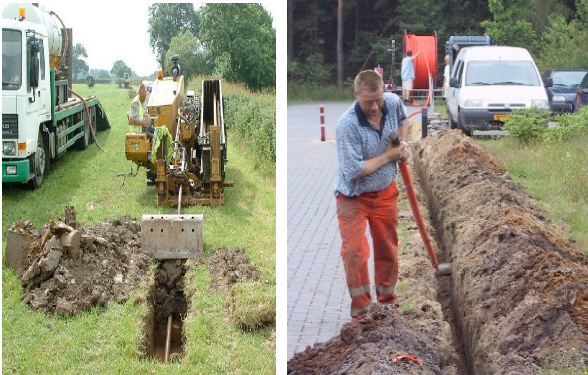
Figure S4: Fibre being installed at JBO (2004) and JIVE (2002).
