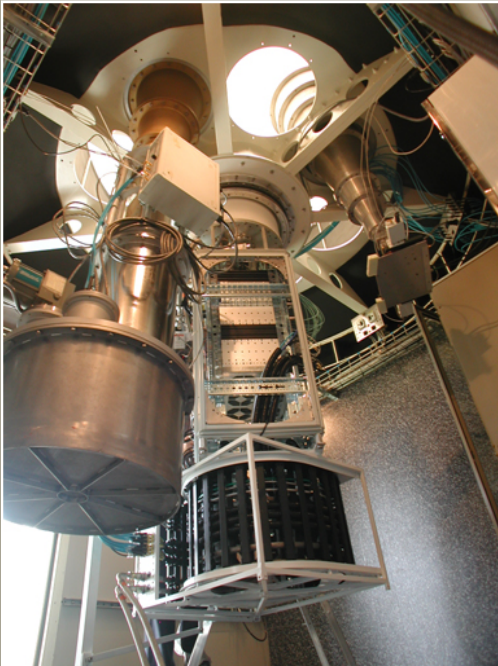
Figure: 18-26GHz Multifeed system (central location)
