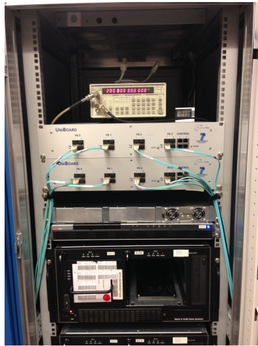
Fig. 3.6 EVN next generation correlator: two UniBoard units with clock generator and power supply
