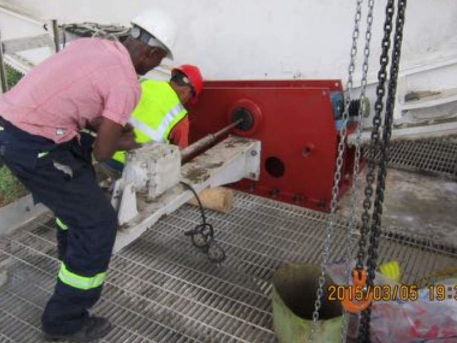
Ghana (March 2015) replacing shock absorbers, stow pin brackets, stow pins, limit switches
