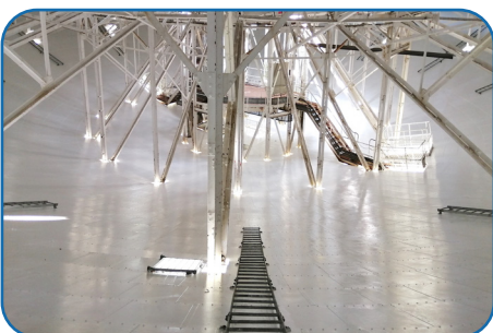
A new surface for the Lovell 76m radio telescope in Jodrell Bank
